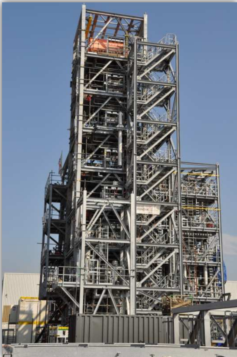
Picture of the plant structure front side
