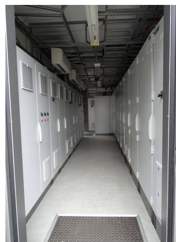
Control interface & power distribution cabinet
